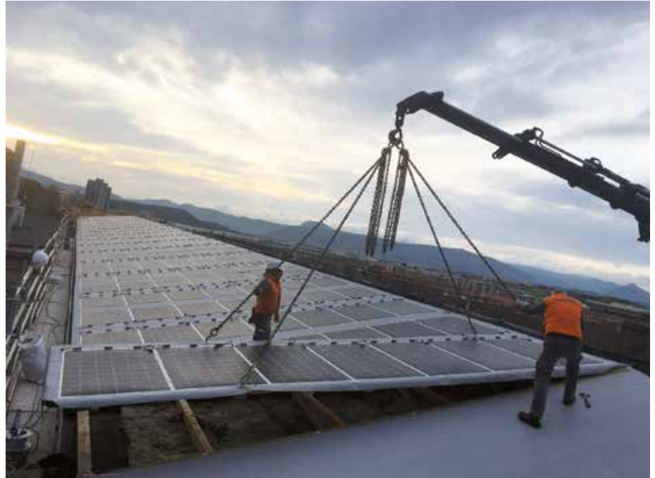
Figure 1: Installation of a prototype Plug&Play solar roof on the Municipal Police building in Pamplona (Spain). The panels will provide energy for self-consumption and are connected to recycled batteries for energy storage
