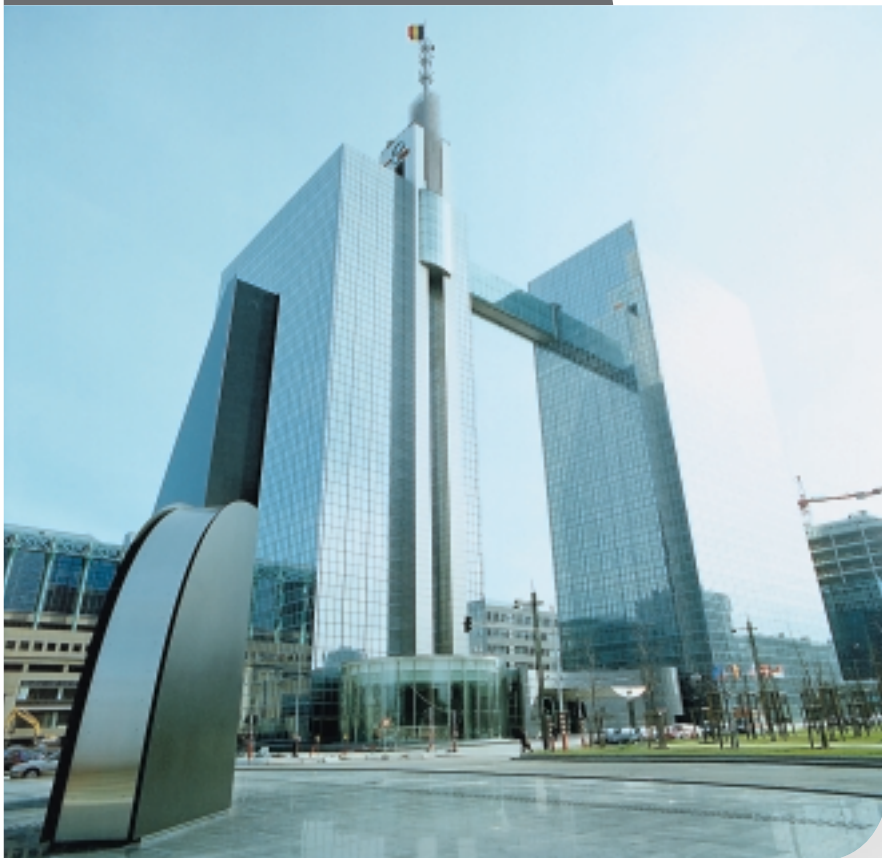
The Belgacom Towers in the heart of Brussels
