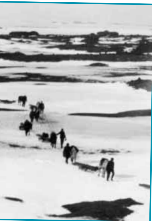
Horses pulling telephone poles in 1905
